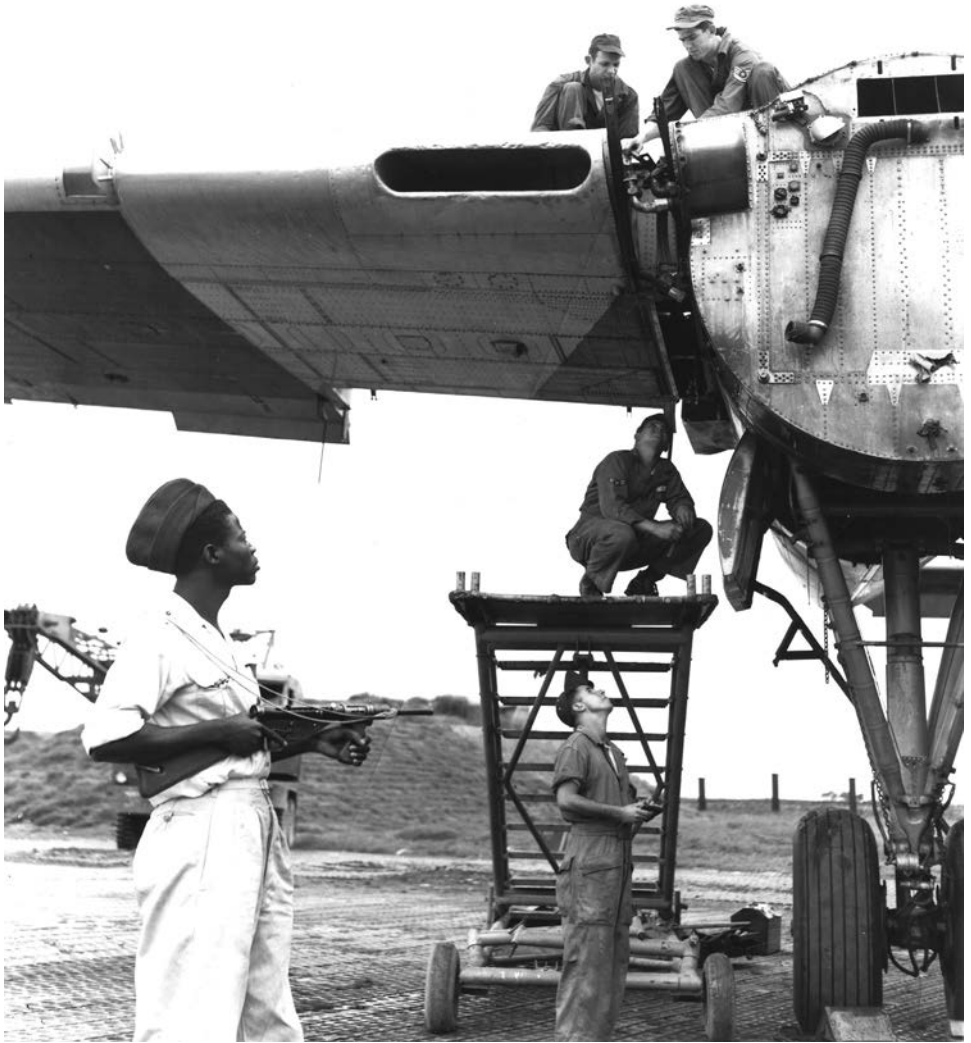
USAF mechanics from the 483d Troop Carrier Wing repair a C-119 at Cat Bi in May 1954 that had been damaged over Dien Bien Phu during the final days of the siege. By this point, there were more than 500 USAF airmen in Vietnam. A Senegalese member of the French Foreign Legion is guarding the aircraft, indicative of the security concerns about sabotage by that time. As the threat level increased, FEAF moved the USAF detachment from Cat Bi to Da Nang on May 22. USAF.
