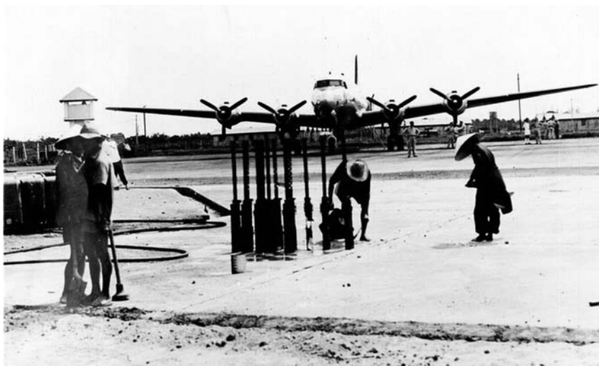
The French employed Viet Minh prisoners to lay concrete for an expanded apron at Tourane (Da Nang). A C-54 from the 374th Troop Carrier Wing is in the background. USAF .
